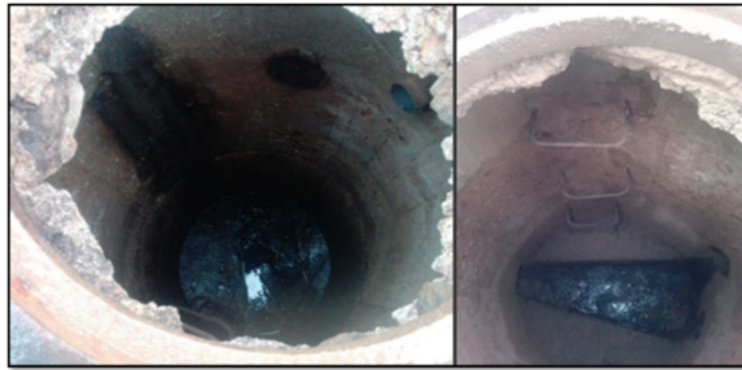
Figure 6. Interior condition of the old sewer inspection wells.
